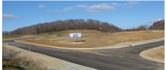
Infrastructure improvements in Gateway Commerce Park
