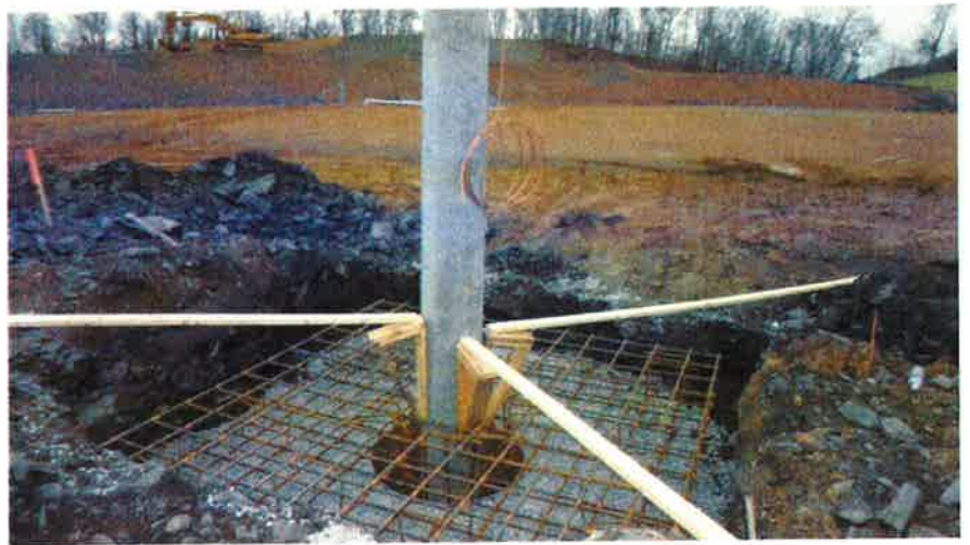
Light Pole Base Between Field 2 & 3 Ready to Pour. Note Perimeter Pole Ready to Stand Up in the Background
