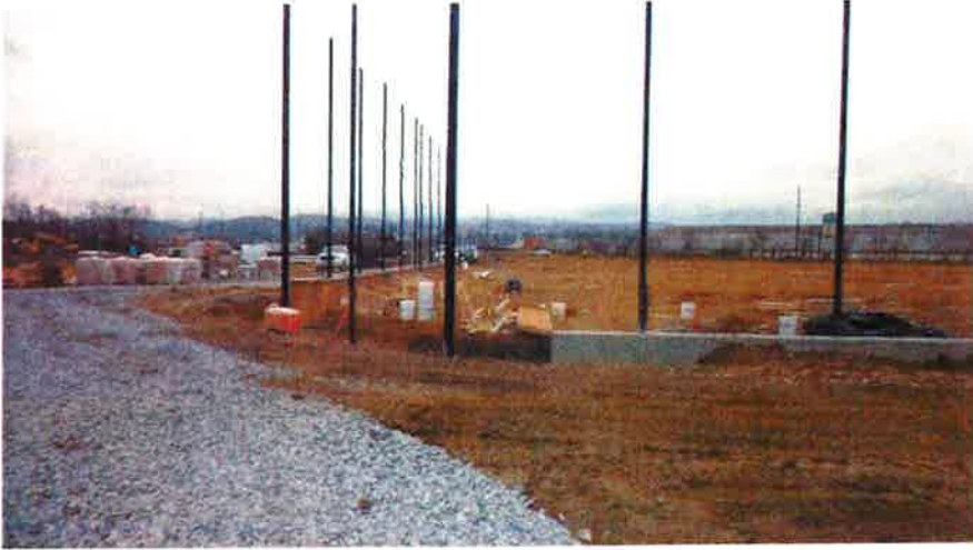
Light Pole Base Between Field 2 & 3 Ready to Pour. Note Perimeter Pole Ready to Stand Up in the Background
