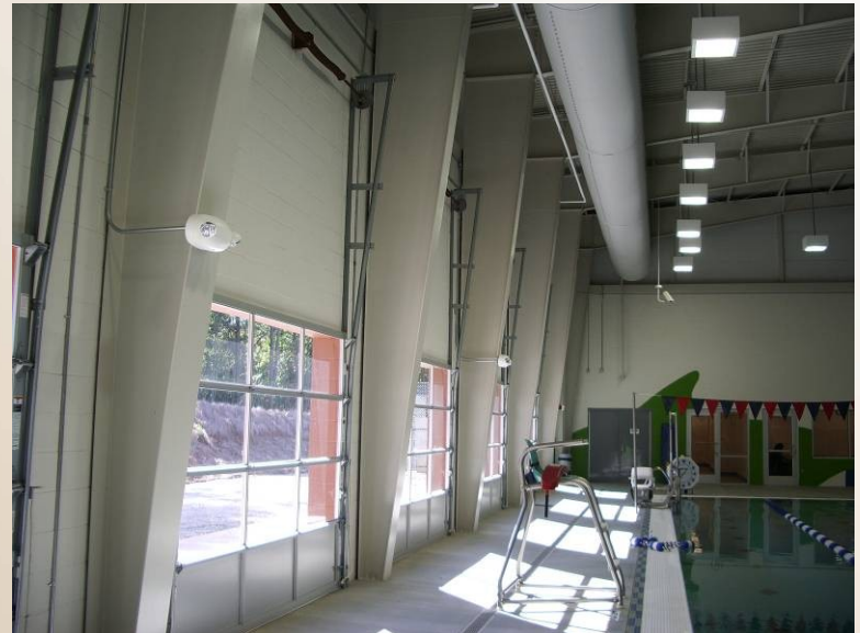
Sliding Glass Panel Doors Between Pools
