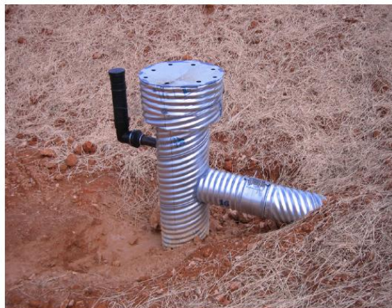
Figure 7.31-6 Dewatering device on Riser with Trash Rack
