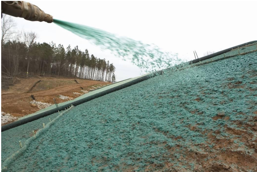
Hydraulically applied seed, mulch and binder
