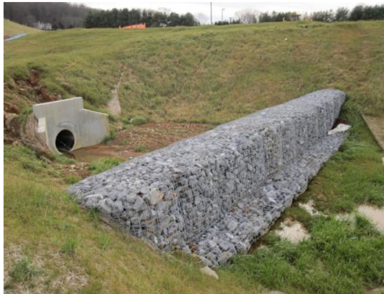
Figure 7.31-2C Forebay with Porous Berm (Gabion Rock)
