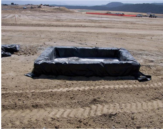
CONCRETE WASHOUT
