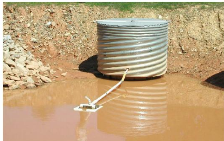
Figure 7.31-10B Floating Skimmer Installation
