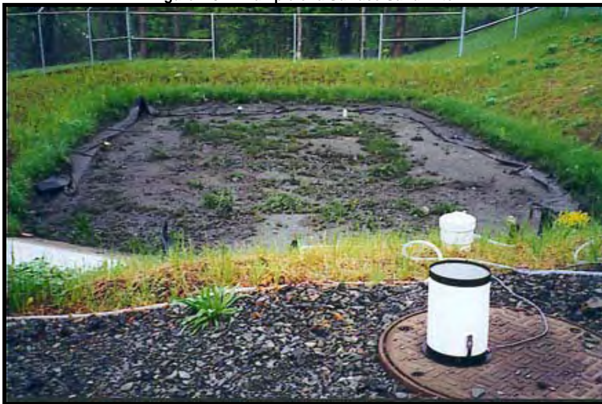
Figure 4-31. Example of a Surface Sand Filter
