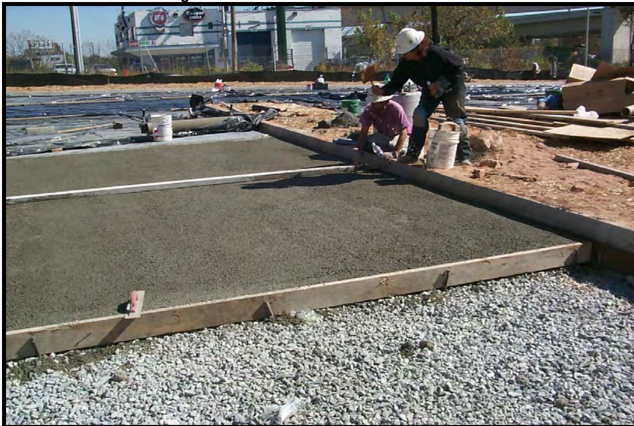
Figure 4-54. Porous Pavement Installation
