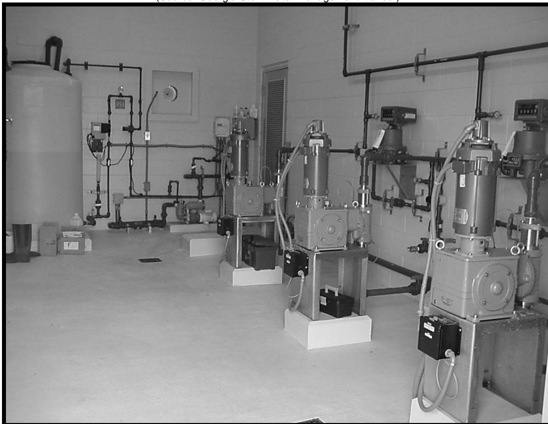
Figure 4-67. Dosing/Injection Components of an Alum Treatment System
