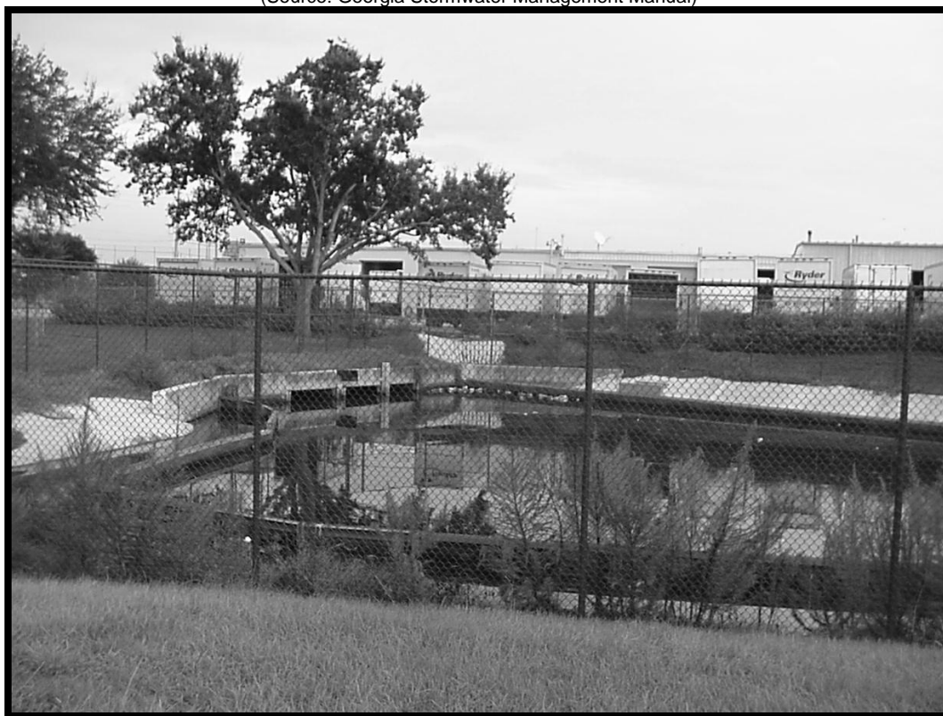
Figure 4-66. Settling Basin for an Alum Treatment System
