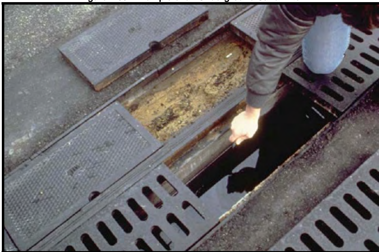
Figure 4-59. Example of an Underground Sand Filter
