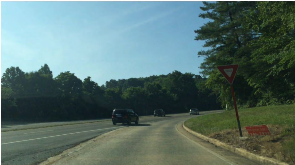
(LM 10.55) SR 93 looking south at on-ramp at end of project.
