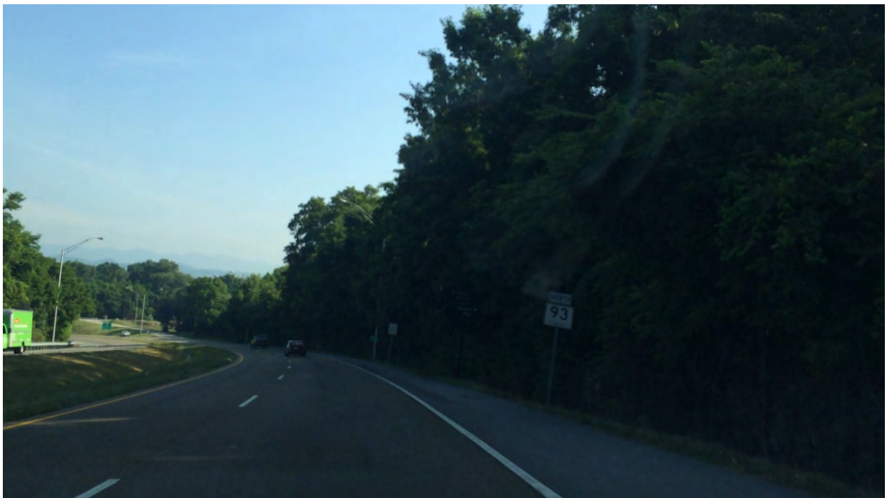
(LM 10.41) SR 93 looking north along horizontal curve.
