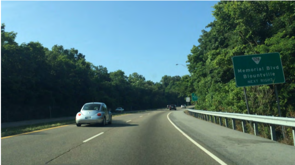
(LM 10.41) SR 93 looking south along horizontal curve.
