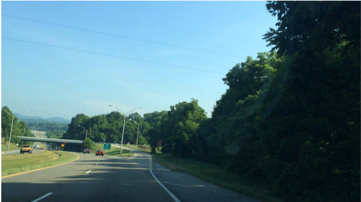
(LM 10.55) SR 93 looking north at off-ramp at end of project.
