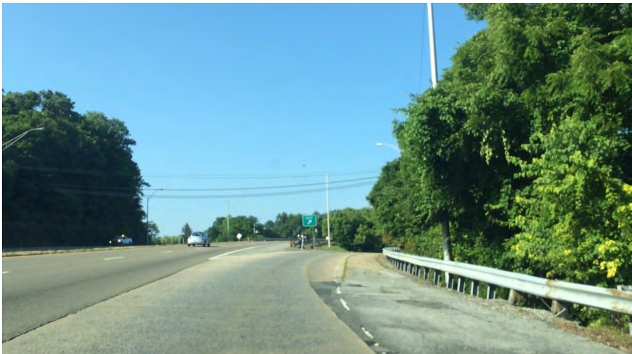
(LM 10.30) SR 93 looking south at off-ramp at beginning of project.
