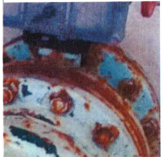
Off Gas of Chlorine from Clearwell
