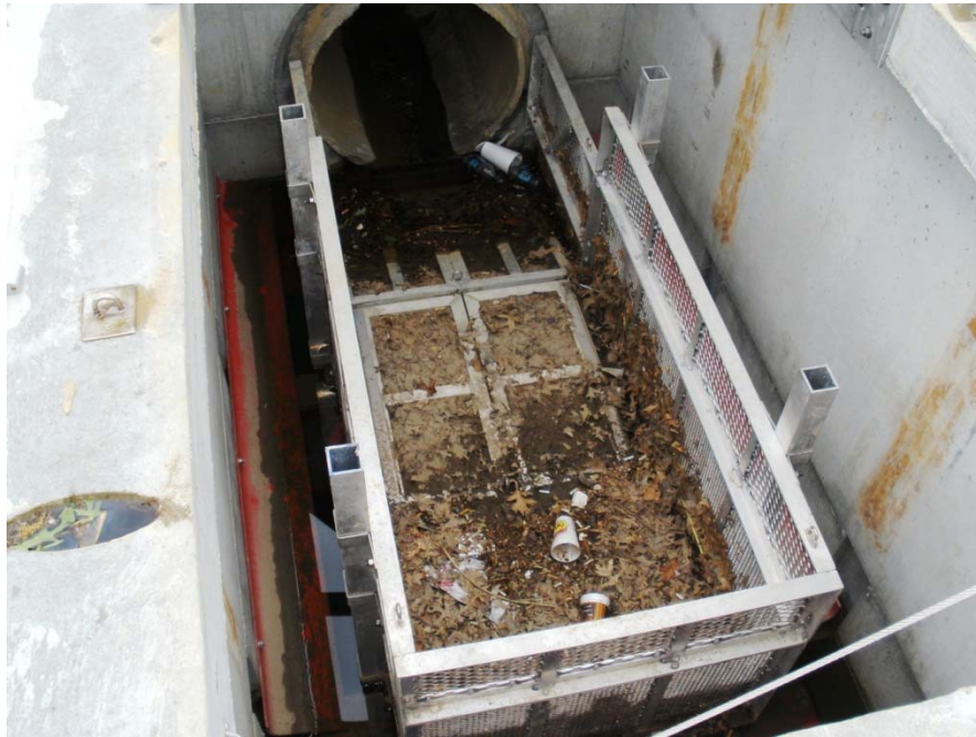
This filtration device along Madd Branch helps keep littered debris out of our water supply
