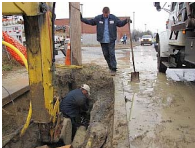
Workers replace a section of pipe
