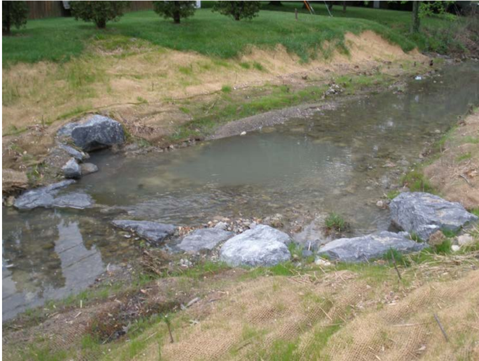
Properly placed boulders can dramatically change the water flow and water quality of a stream
