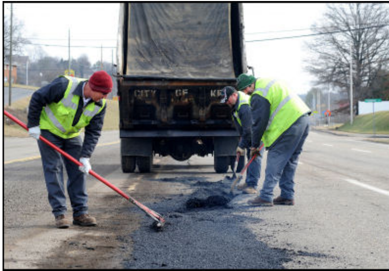
The Street Maintenance crew patches some road damage
