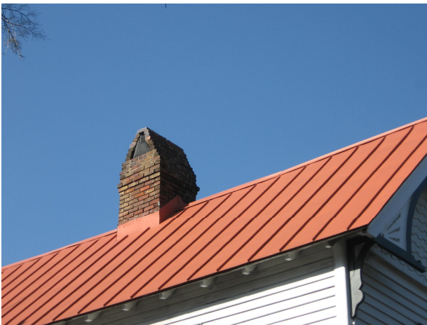
New metal roofs should have appropriate spacing and crimping consistent with historic designs as shown at left.
