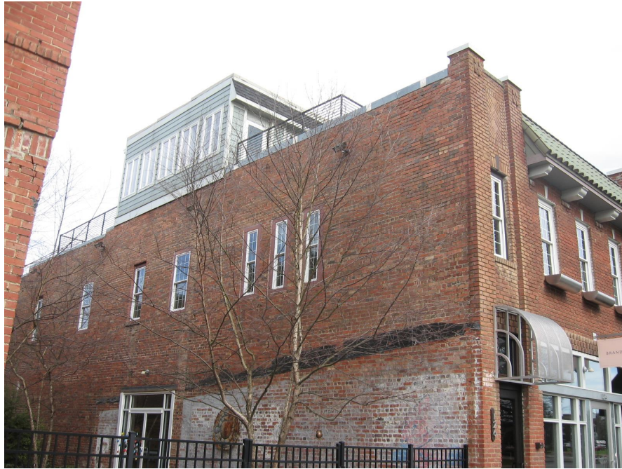
This rooftop addition at 126 W. Main Street is recessed from the main façade and has limited visibility from the street level.
