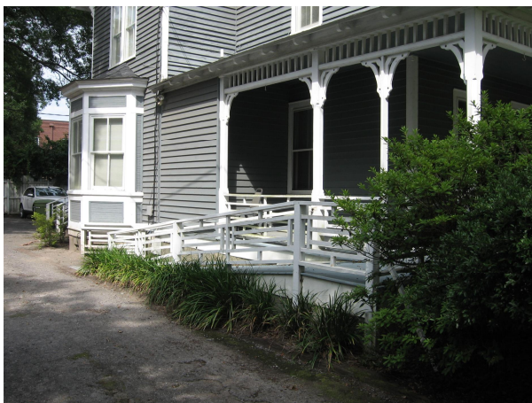
Above and below are examples of appropriately designed ADA compliant ramps on side elevations.
