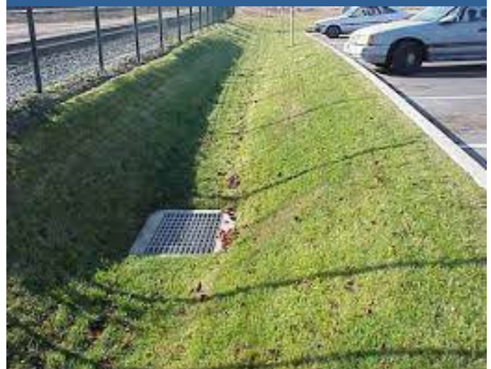
Figure 1. Grass Channel (Source: Nashville LID Manual)
