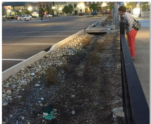
Figure 10. The Importance of Plant Care Poor plant care in this bioretention SCM led to a large repair to remove and replace unhealthy soil and plants.
