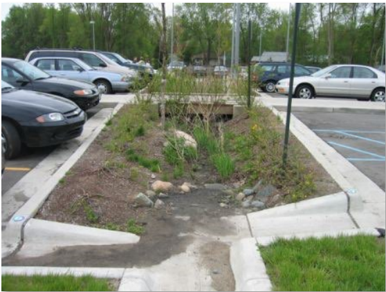
Figure 13. Sediment Disposal The accumulated sediment in this office park bioretention SCM can be put in the trash or used somewhere else on the property. (Source: ces.org)
