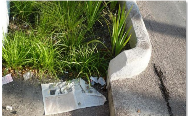
Figure 9. SCM Cleaning Removing trash, leaves, and debris is a routine maintenance activity for all SCMs.
