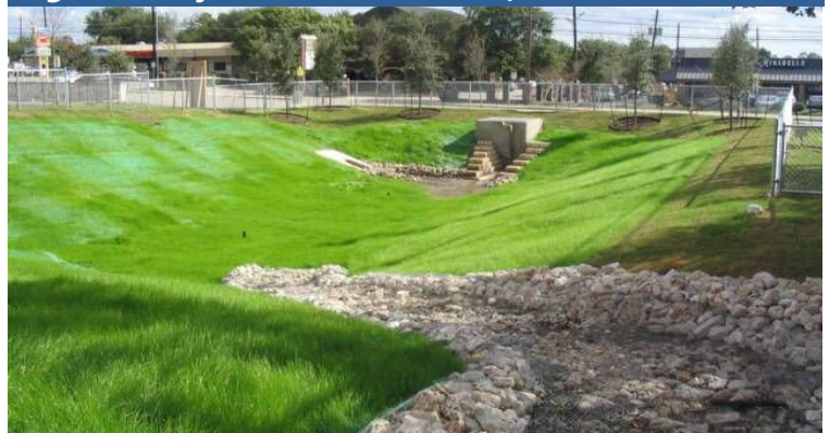
Figure 1. Dry Detention Basin (City of White House TN)
