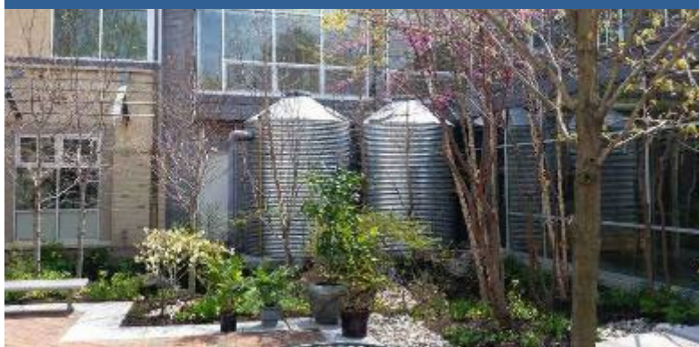
Figure 1. Cistern (Source: Philadelphia Water Department)
