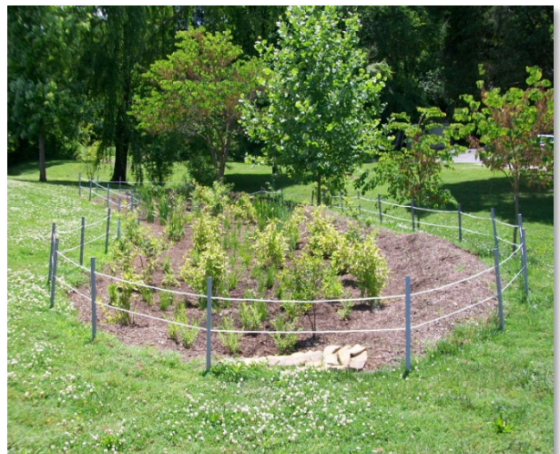
Figure 4. Bioretention SCM. Bioretention SCMs use soil and plants to remove pollutants from stormwater. They are not designed prevent flooding during large storms. (Source: Knox County TN)
