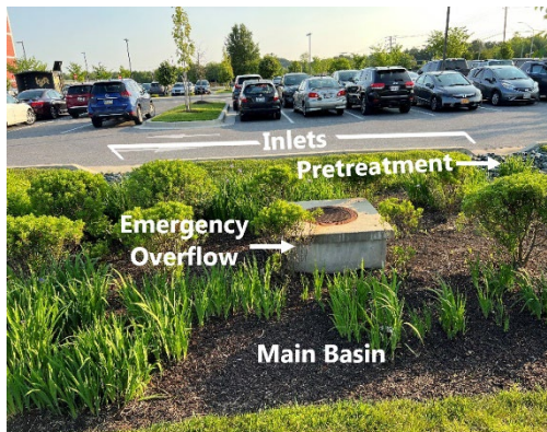
Figure 3. Bioretention Component Examples
