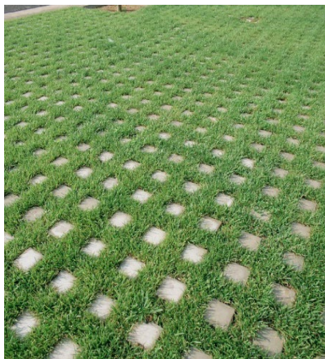
Figure 3. Examples of Different Permeable Pavement Systems Left: Grassed concrete grid pavers (Source: Checker Block® pavers from Nicolock); Middle: Xeripave Super Pervious Pavers (Source: Xeripave LLC); Right: Comparison of porous asphalt with standard asphalt (Source: Virginia Asphalt Association)
