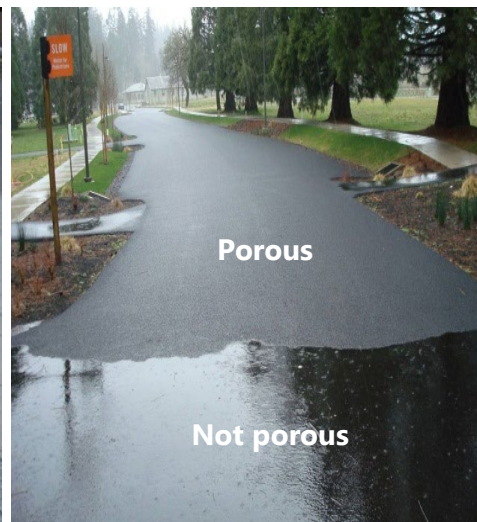
Figure 3. Examples of Different Permeable Pavement Systems Left: Grassed concrete grid pavers (Source: Checker Block® pavers from Nicolock); Middle: Xeripave Super Pervious Pavers (Source: Xeripave LLC); Right: Comparison of porous asphalt with standard asphalt (Source: Virginia Asphalt Association)
