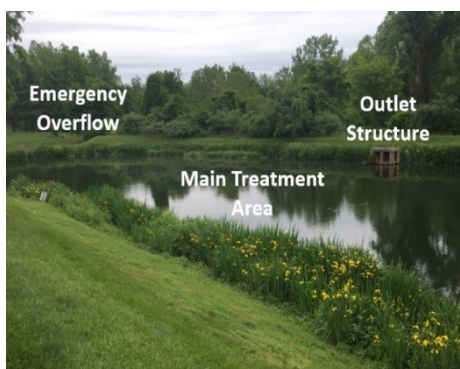
Figure 3. Water Quality Basin Components.
