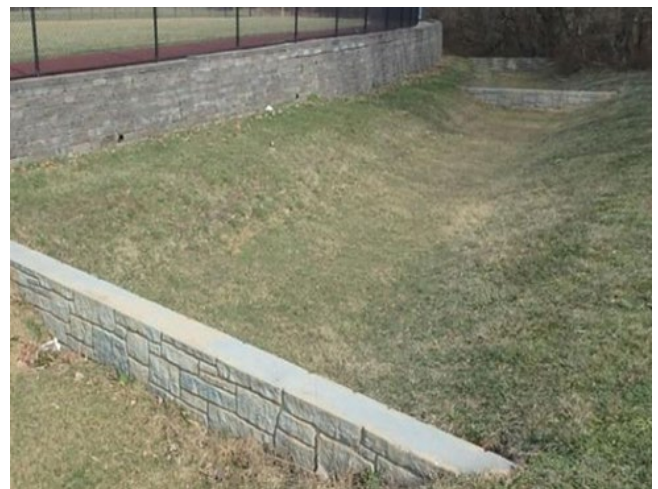
Figure 1. Dry Enhanced Swale The low concrete check dams slow stormwater, allowing runoff from small storms to soak into the soil. During large storms, runoff flows safely over the dams and continues downstream. (Source: MD Dept of Environment )
