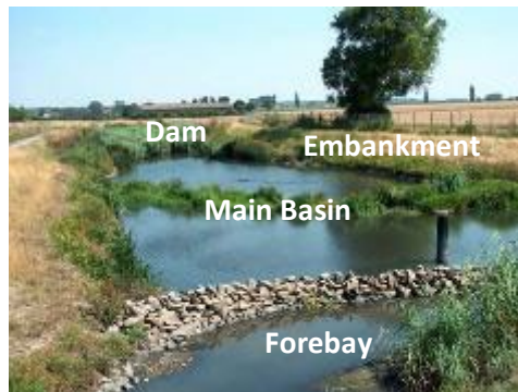
Figure 3. Stormwater Wetland Components Wetland plants are critical to removing pollutants in a stormwater wetland. To keep plants thriving, forebays are important features because they capture trash, debris, and heavy sediments before the water flows into the main basin. (Left: Dragonfly Pond Works; Right: www.constructedwetlands.com)
