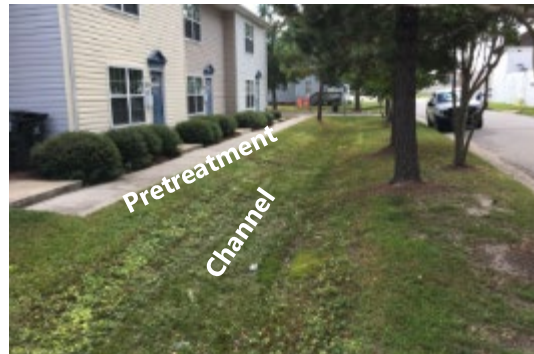
Figure 3. Grass Channel Components
