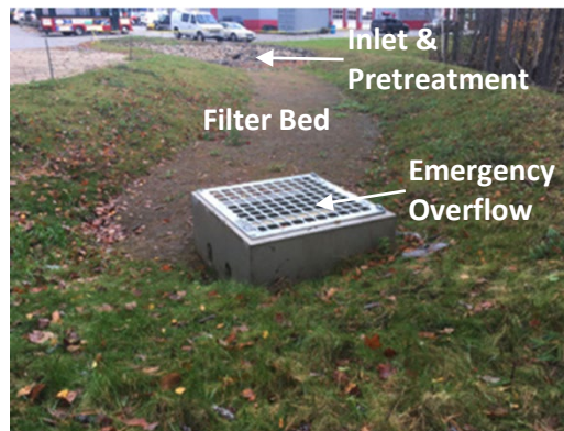
Figure 3. Examples of Sand Filter Components
