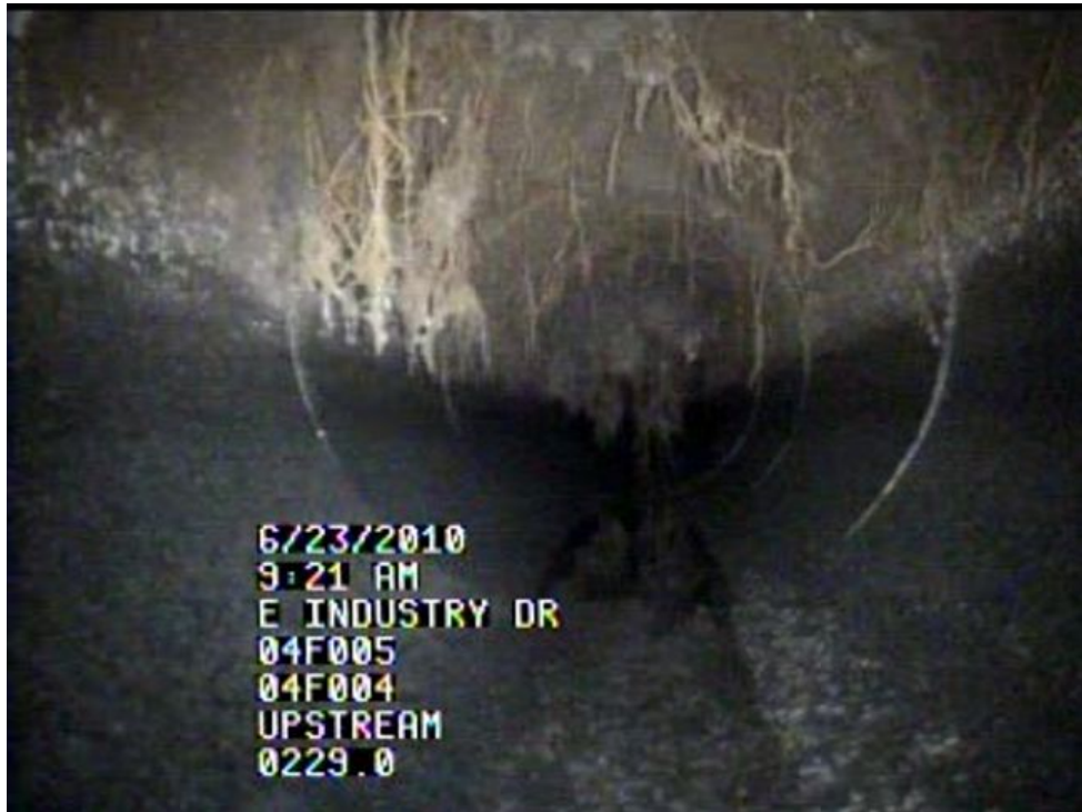
Industry Drive Sewer Line (Pre-Cleaning)
