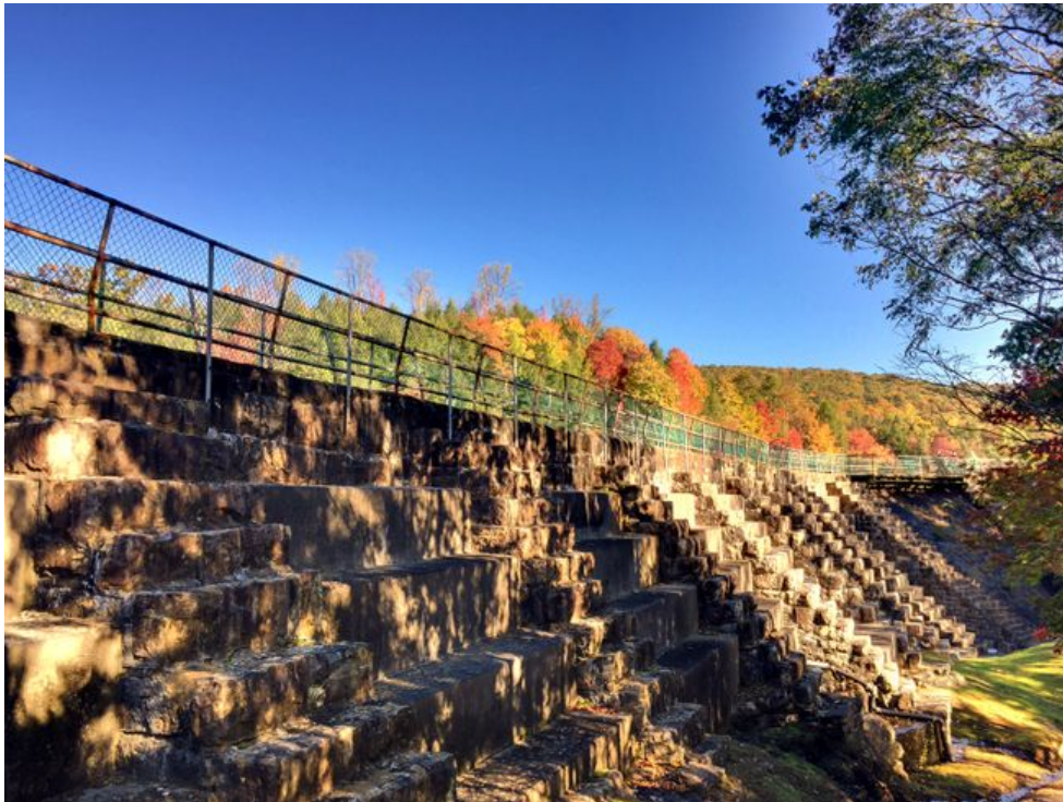
Bays Mountain Dam
