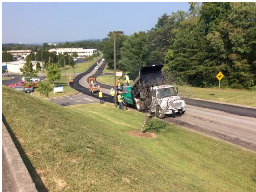
Street Maintenance Crews paving area roads
