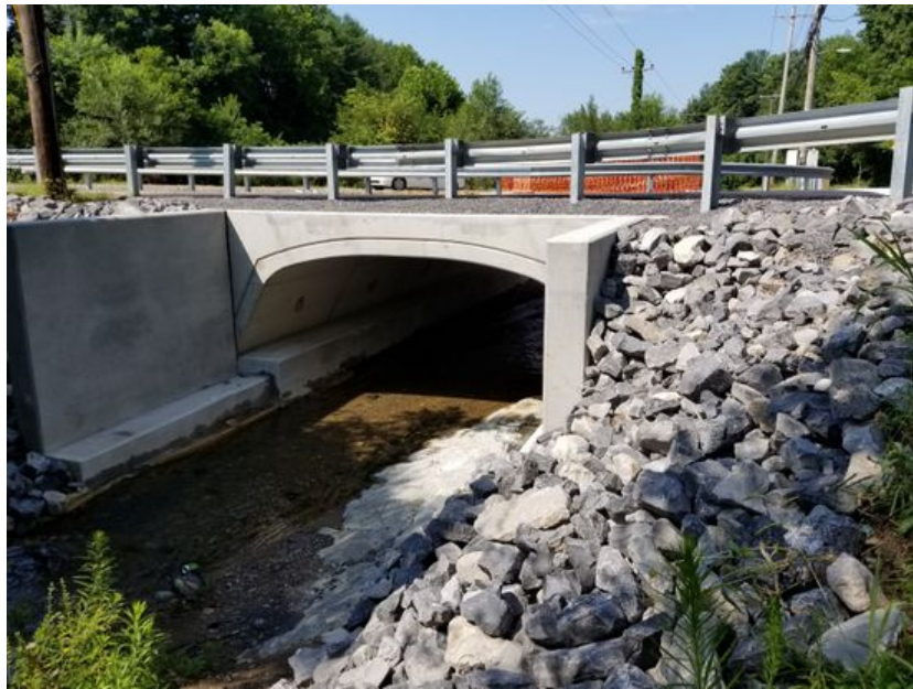
Replacement of a failing culvert crossing on Bloomington Drive
