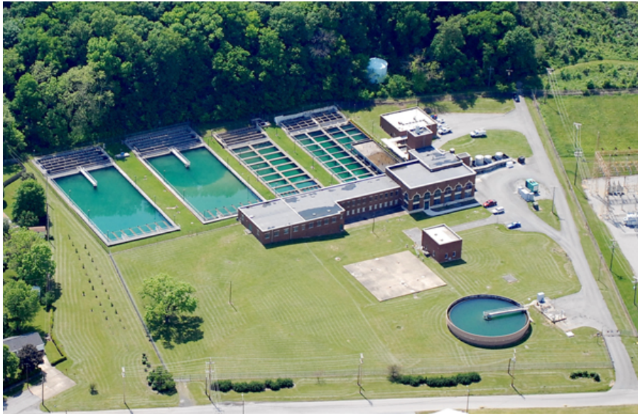
Aerial view of the Kingsport Water Filtration Plant
