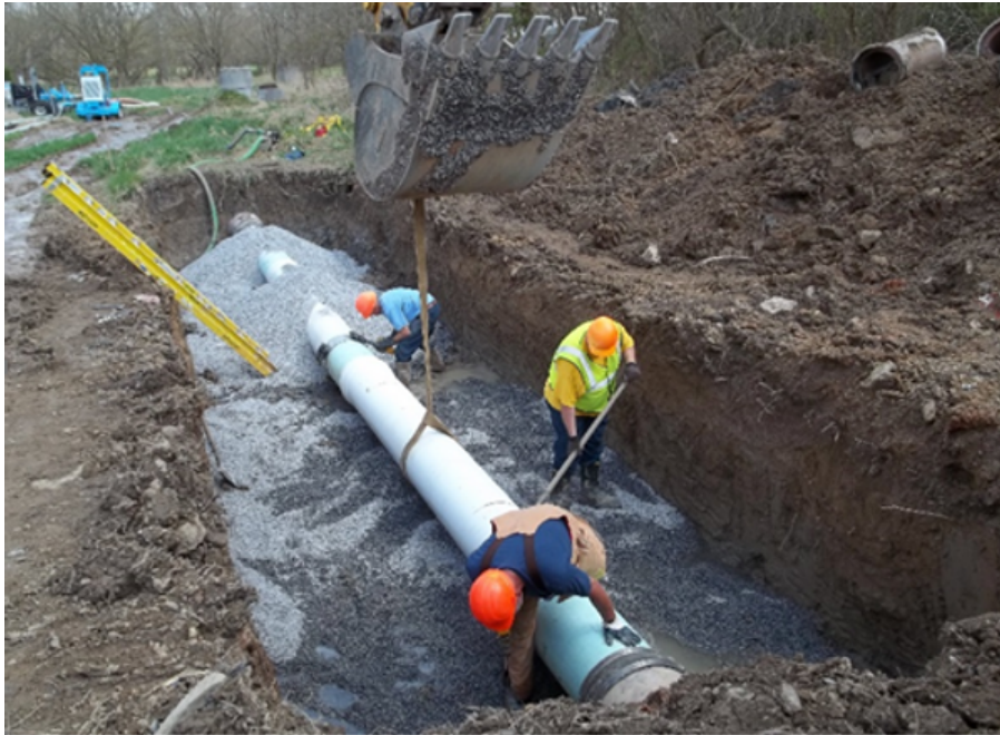
Wastewater Maintenance Crew in the field
