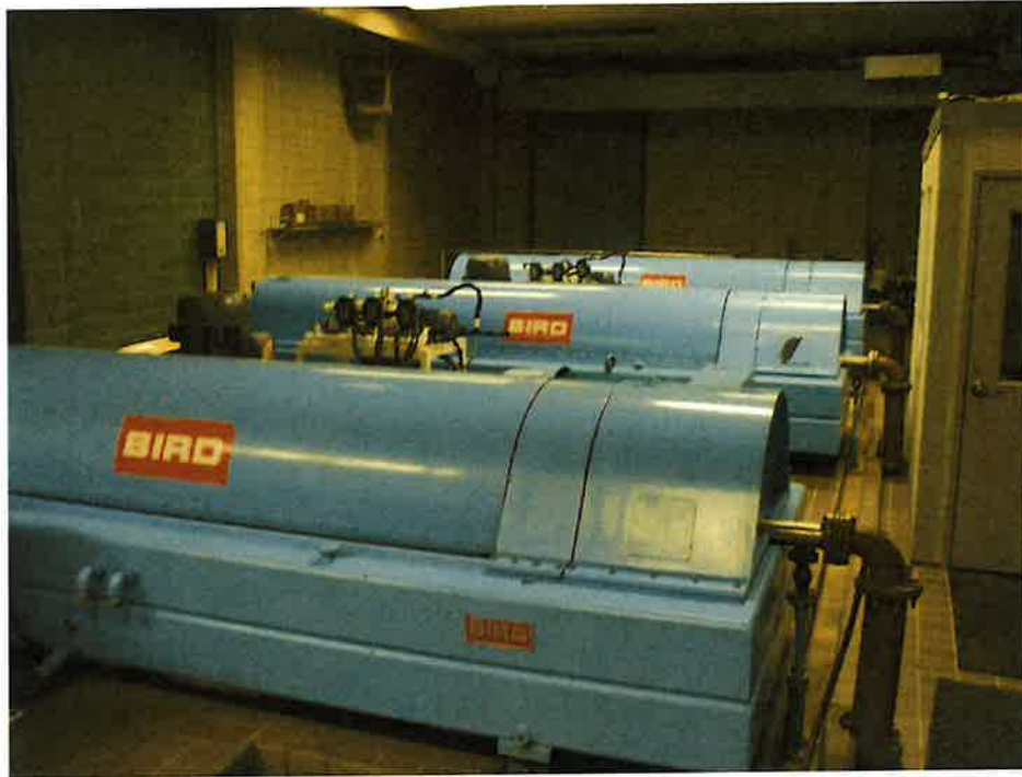
Centrifuge #1 Out of Service
