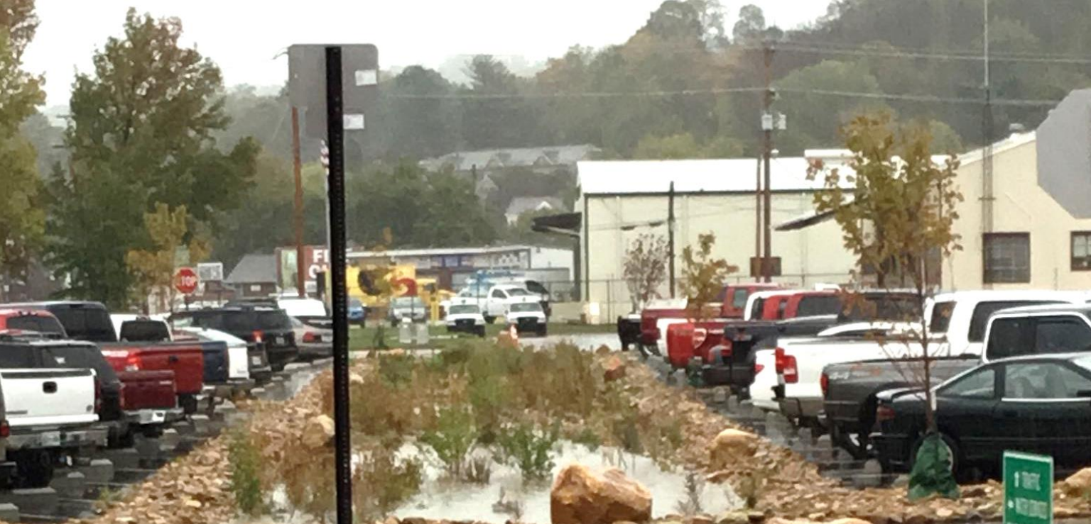
A bioretention area, like the one at Water Services, is a shallow and landscaped depression that receives runoff from impervious surfaces. These areas are often referred to as rain gardens.
