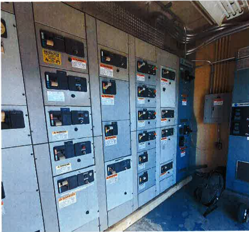
Motor Control Center (MCC) 6 – Installed in 1980 and single point of failure for critical process
