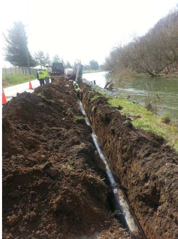
Waterline Replacement on Riverport Rd
