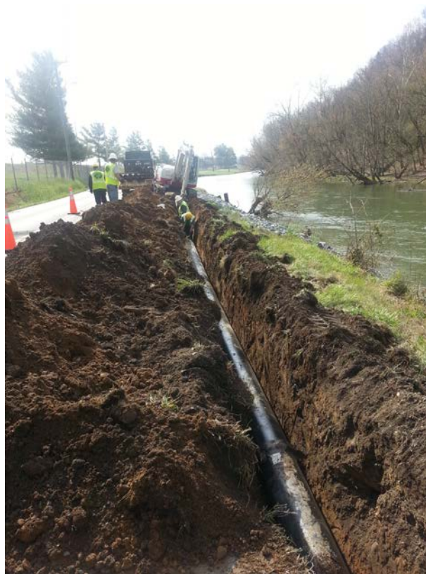
Waterline Replacement on Riverport Rd
